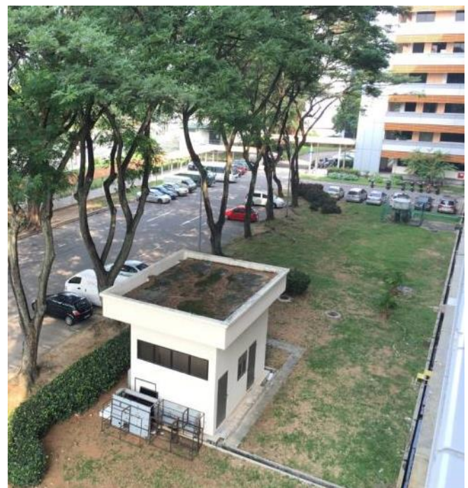
Development of Hi-Tech Building at existing car park
